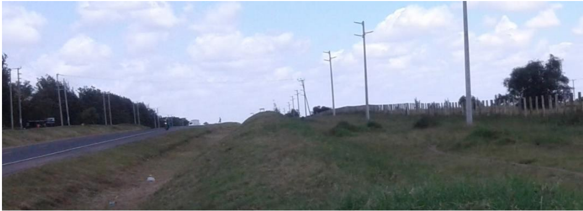
Figure 3-73: Electricity lines connecting electricity along Namanga-Nairobi highway
