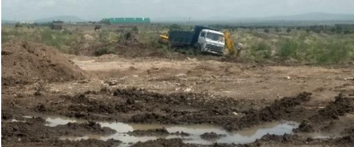
Figure 3-17: Lorry being loaded in a Murram quarry in Milimani
