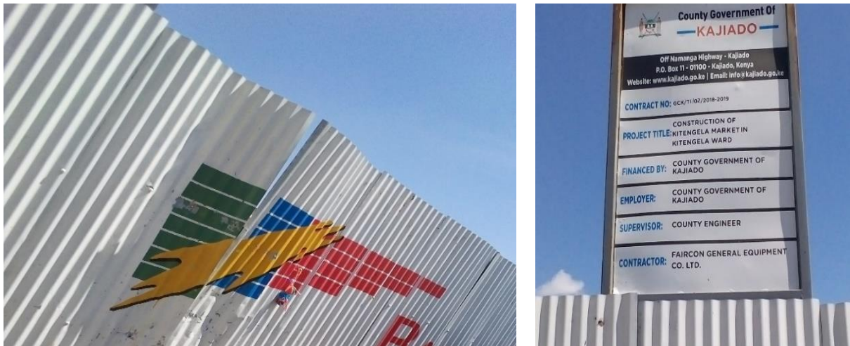
Figure 3-35: Main market construction site
