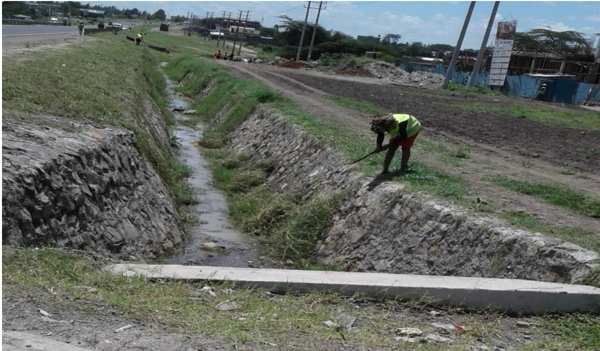
Figure 3-81: A well-constructed storm water drainage outside Riverine estate
