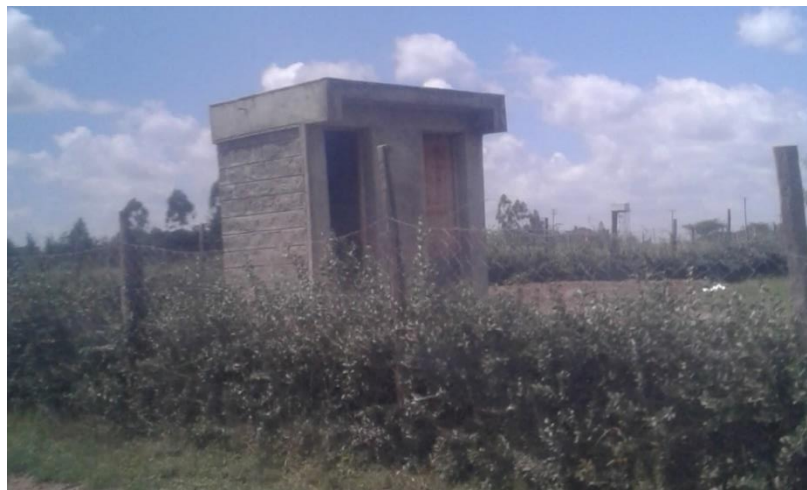
Figure 3-76: A ventilated improved latrine
